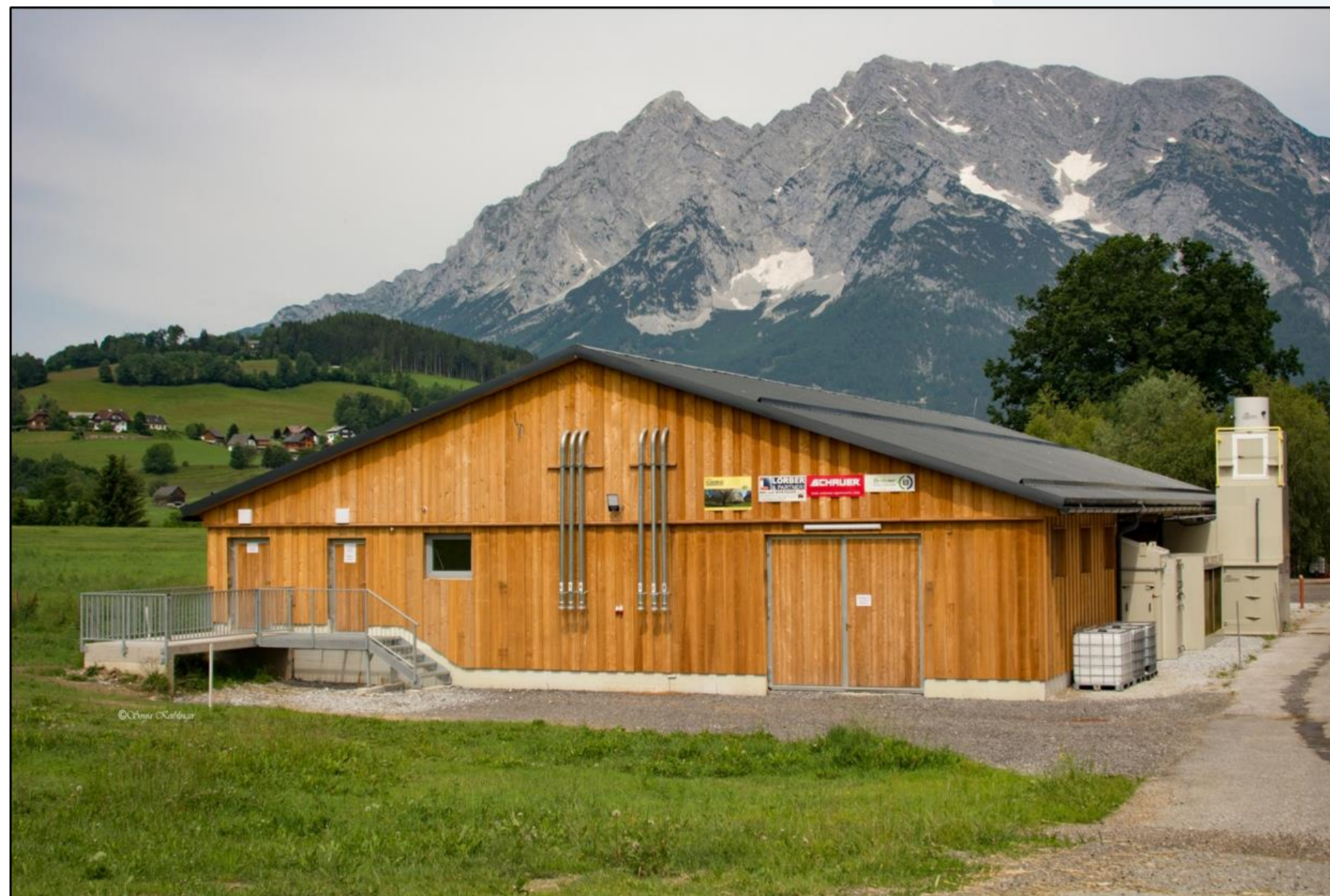
Abb. 1: Pig Research Stable HBLFA Raumberg-Gumpenstein with air purification equipment on the right side of the building.
