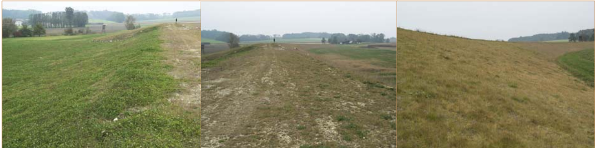
Figure 12: Three different views on the flood detention basin in Stillbach. The first view is on immature soil with the seed mixture ReNatura AV2. The second view is on top of the dam where lanes from cars and vegetation are visible. The third view is on Breiningsdorfer and Waldzeller gravel with different seed mixtures AV1 and BM 1
