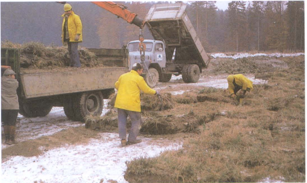
Figure 4. Grass turfs are very suitable for the rapid and site specific restoration of damaged areas.
