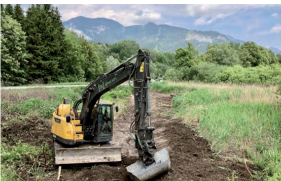
Figure 10 – Clearing and reactivation of drainage ditches. © W. Starz 2018
