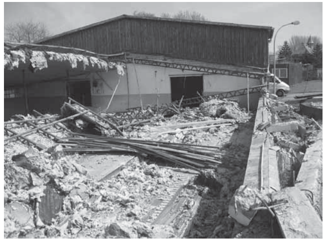
Figure 2.4.2.1.1: demolition of a cattle building: Mixture of old building materials has to be sorted due to contemporary environmental regulations.
